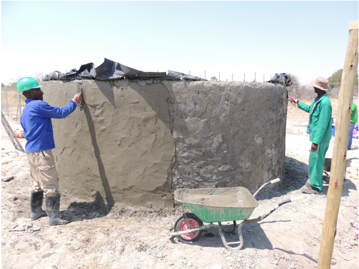
Figure 21: Application of plaster to the outside wall of the ferrocement tank and smoothing of the surface.
