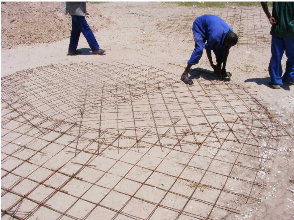
Figure 5: Cutting reinforcement mesh for foundation into circular shape.
