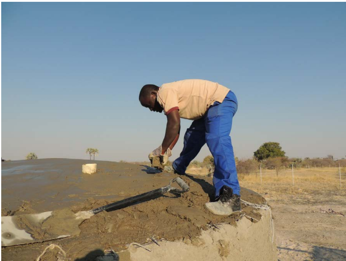
Figure 28: Application of mortar to the roof reinforcement and smoothening of the surface with wood float.
