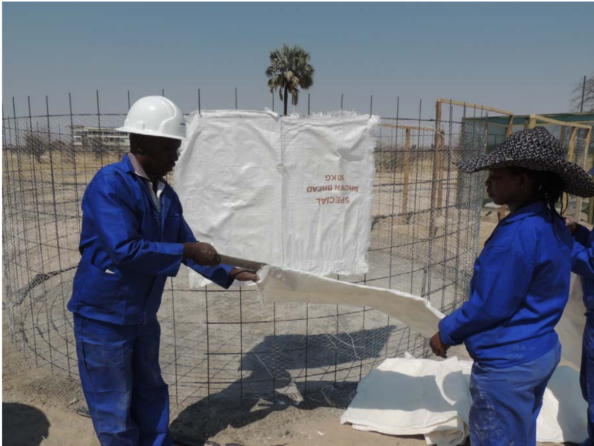
Figure 11: Placing sacks to sidewall reinforcement (already covered with chicken mesh) from the outside.
