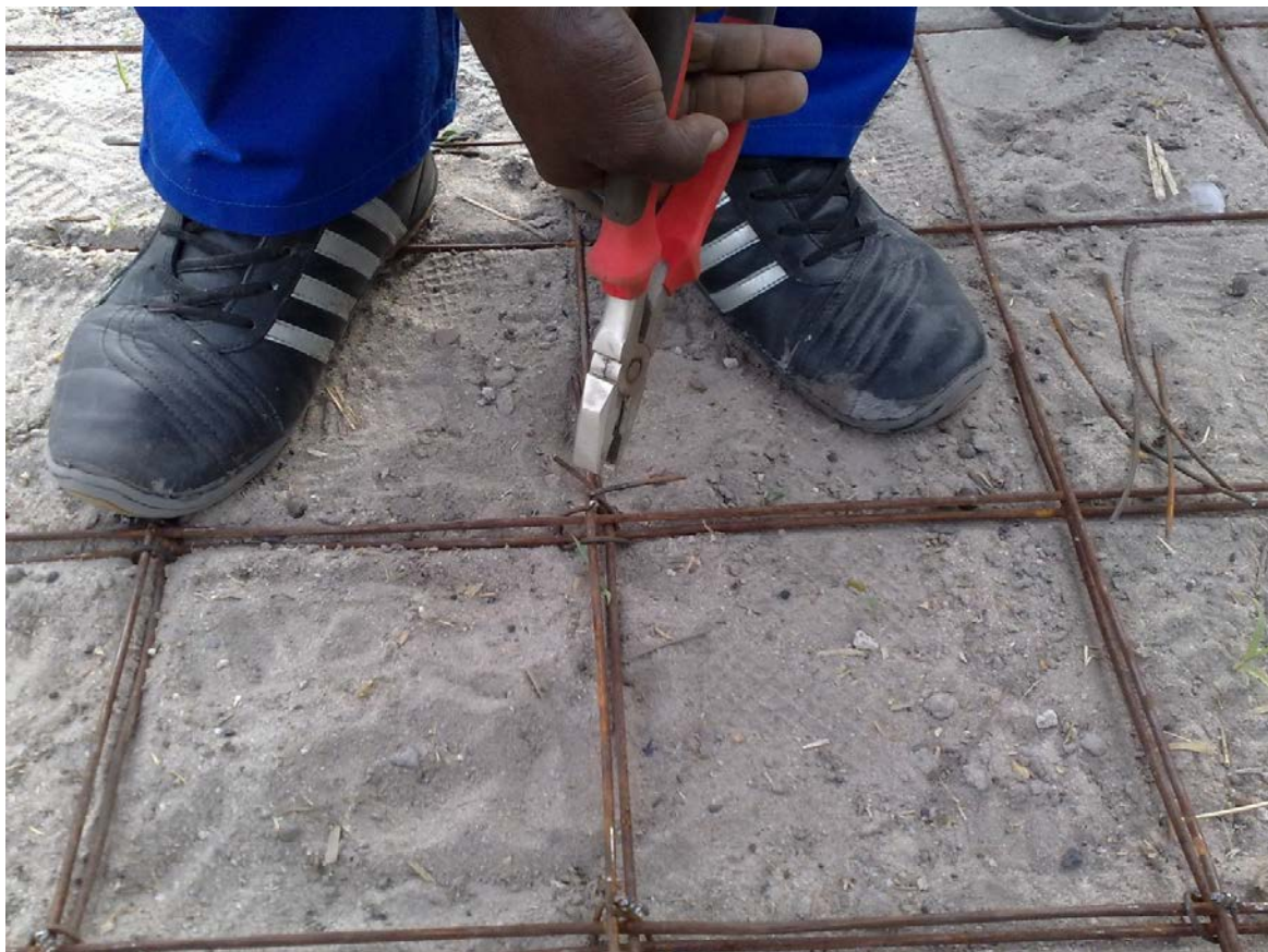
Figure 4: Usage of binding wire to tie reinforcement steel together.
