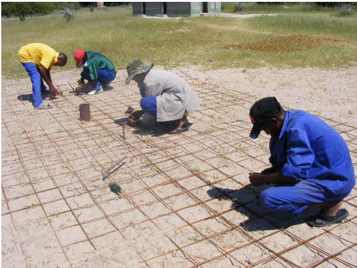
Figure 3: Tying reinforcement steel meshes together to build reinforcement for foundation.
