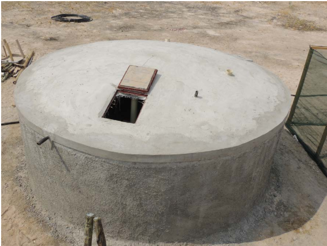
Figure 29: Nearly finished ferrocement tank with overflow pipe (left), manhole cover (centre), and opening for water inlet (upper right side). (The base of the tank is not yet plastered on this picture.)
