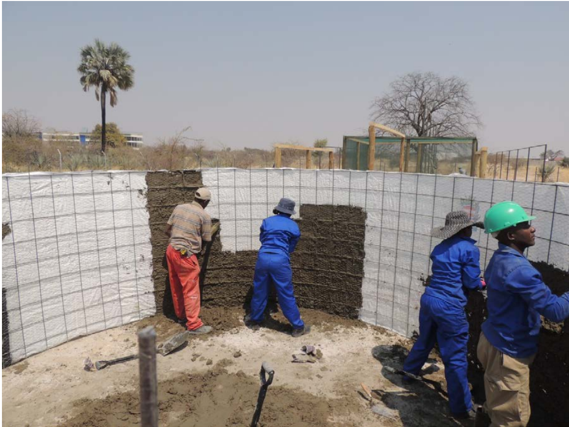
Figure 16: Applying the first layer of plaster to the sidewall from the inside.
