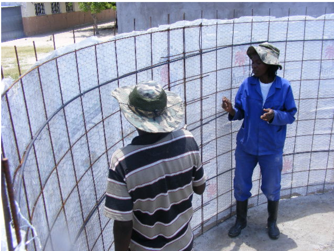
Figure 14: Tying 8mm steel bars to sidewall reinforcement from the inside (from the ground each 40 cm to the top).
