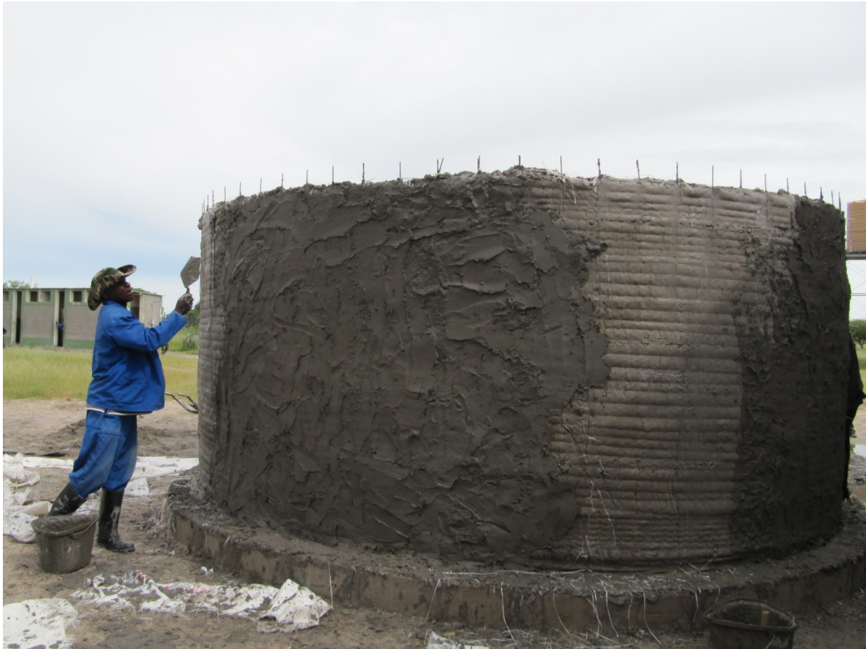
Figure 20: Plastering the sidewall of the ferrocement tank from the outside after removal of sacks.
