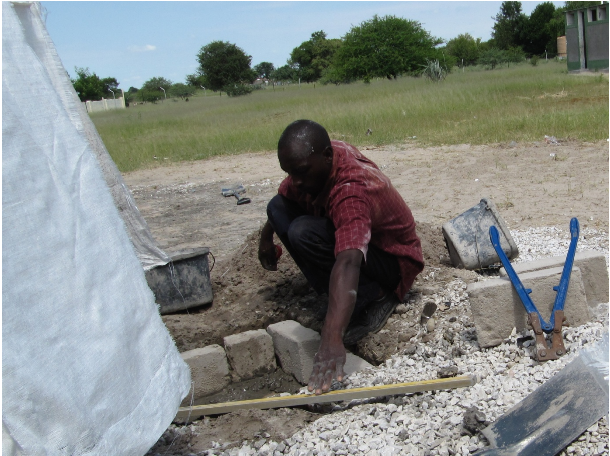
Figure 17: Placing bricks into future water tap pit.
