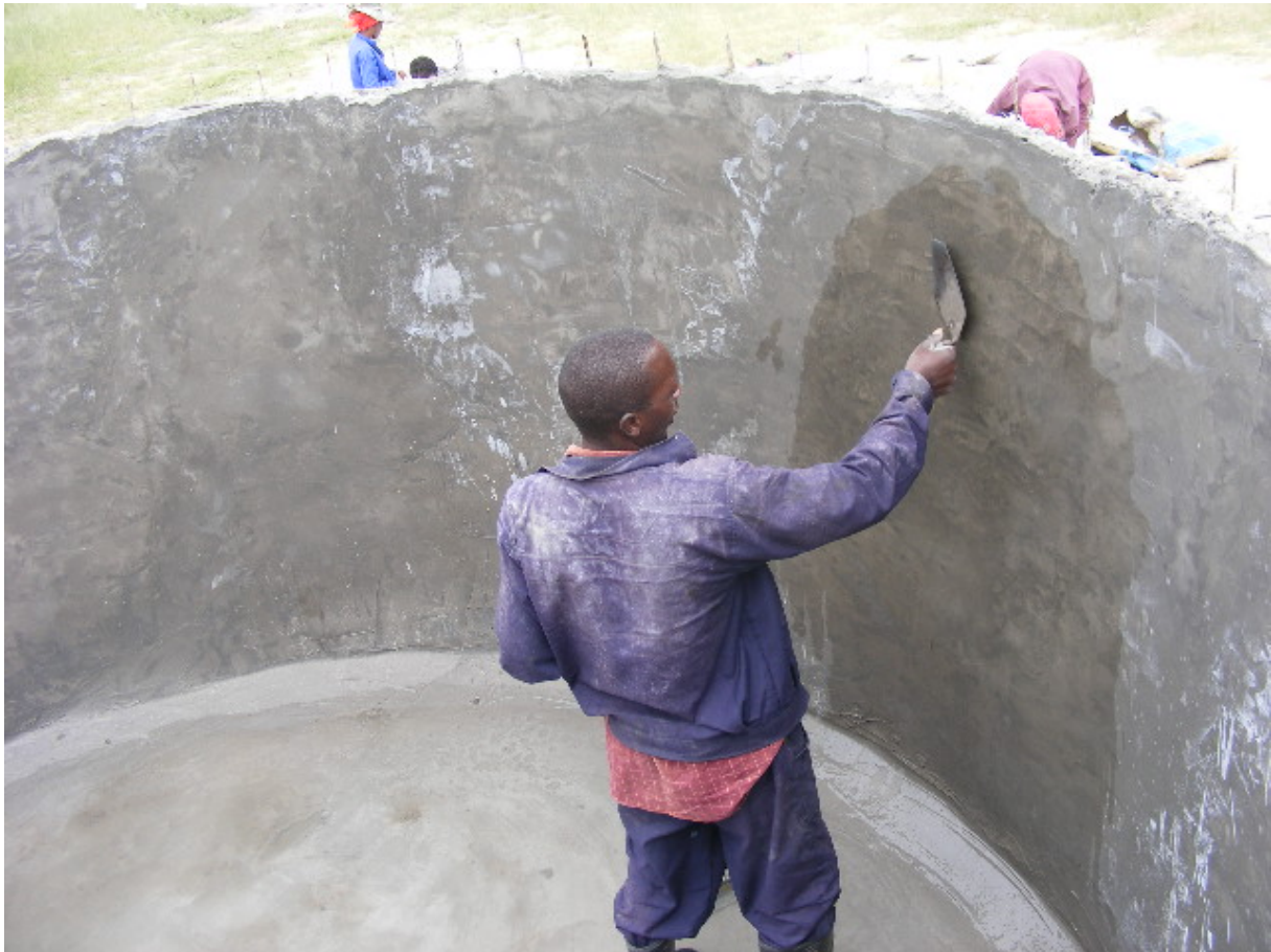
Figure 19: Application of cement slurry (NIL) to sidewall from the inside (floor and edges already smoothed)
