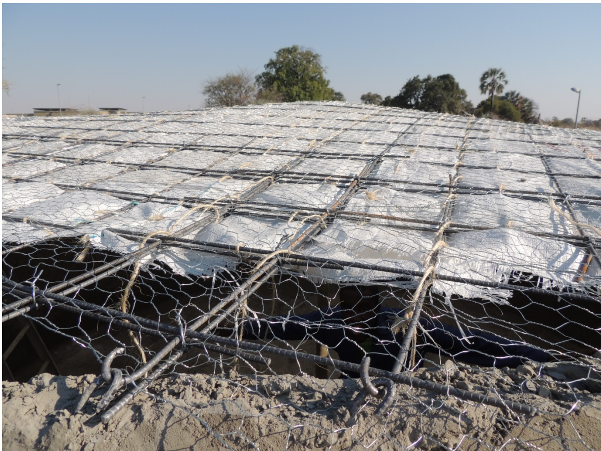
Figure 24: Roof reinforcement fixed tot he sidewall by bending the steel bars and usage of binding wire.
