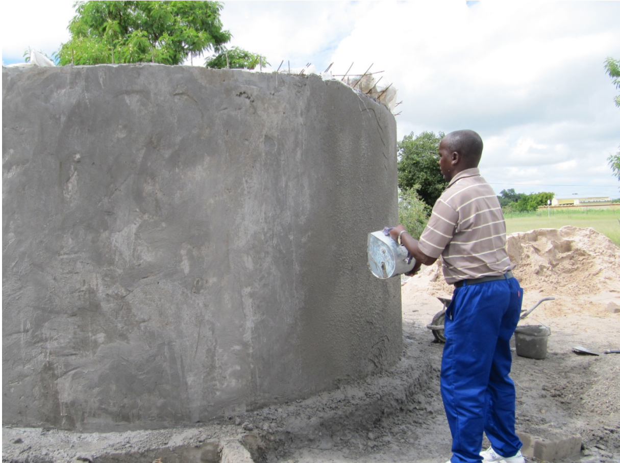
Figure 23: Application of final layer of plaster with plaster sprayer. Border of foundation not leveled and smoothened yet.
