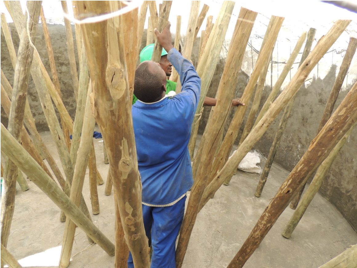
Figure 25: Placing support poles into the tank to support the roof reinforcement and form a dome shape.
