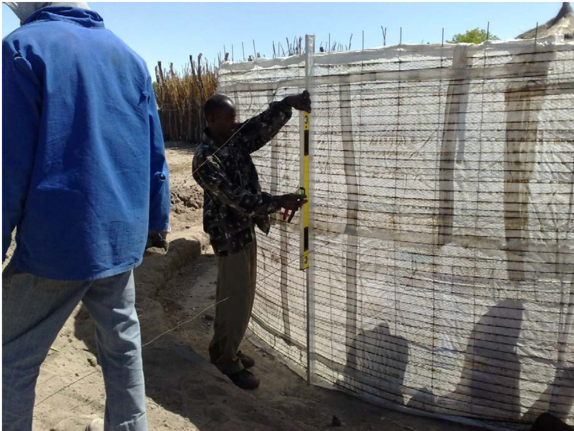
Figure 15: Leveling and fixing sidewall in position.
