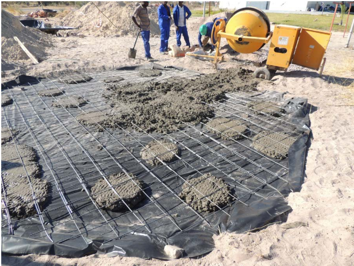
Figure 9: Plastic foil and steel reinforcement for foundation of ferrocement tank.
