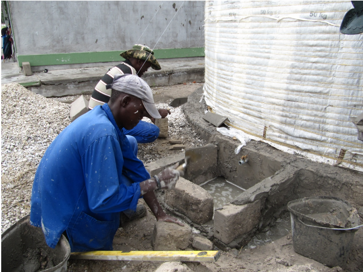
Figure 18: Laying second layer of bricks and plastering the future water tap pit
