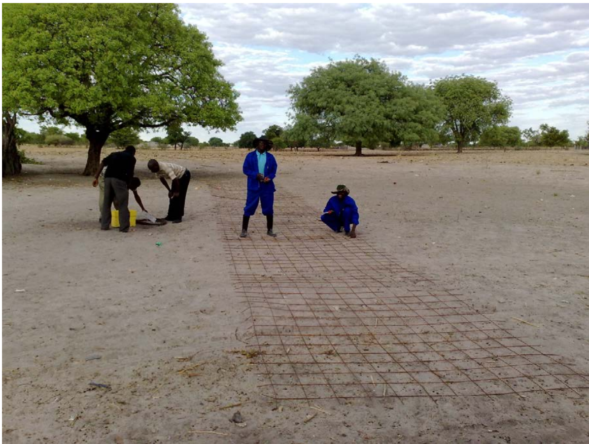
Figure 6: Positioning and tying of steel meshes to a stripe of 14m length.
