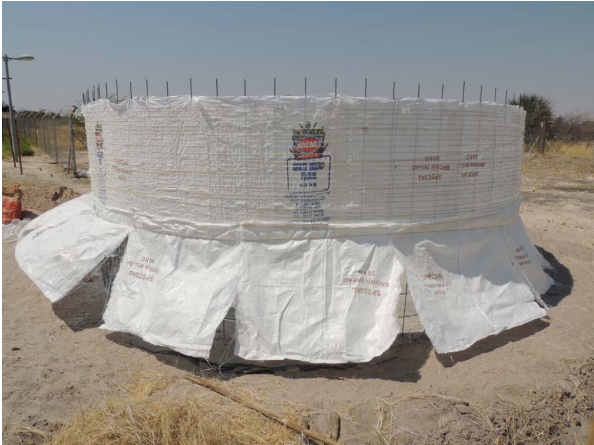
Figure 12: Tying sacks to sidewall reinforcement with cord.
