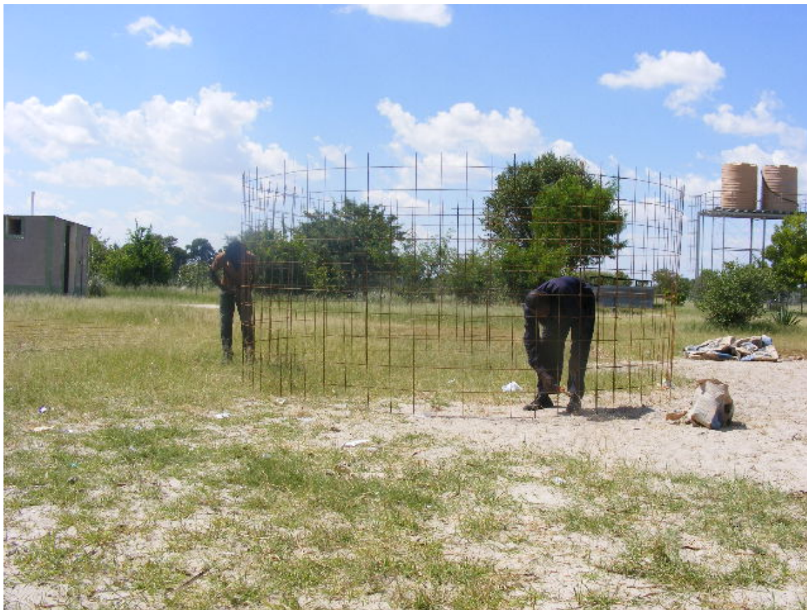
Figure 7: Forming a circular tube with the reinforcement of the sidewall.
