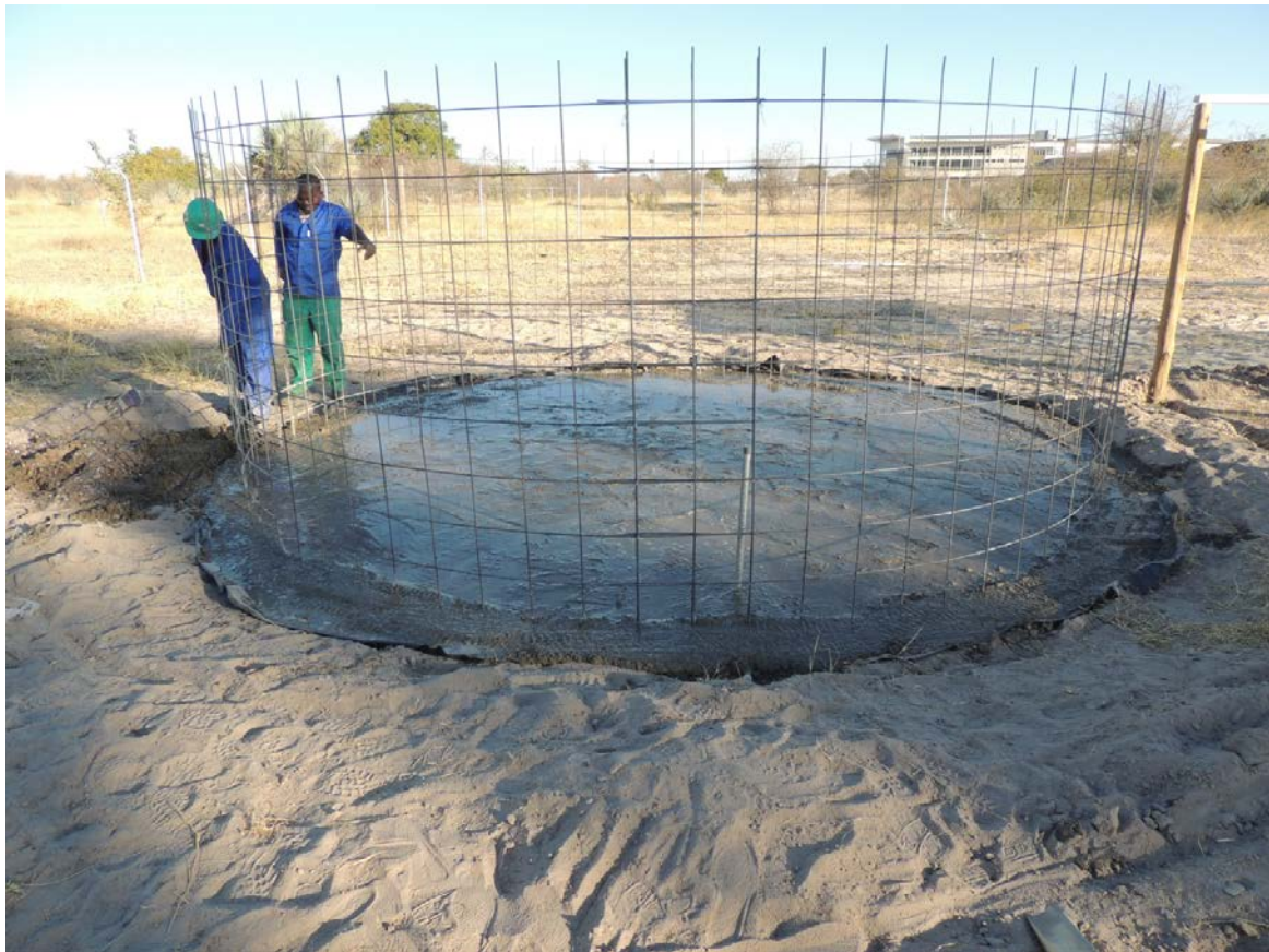
Figure 10: Sidewall reinforcement tied to foundation reinforcement and foundation filled with concrete (draw-off pipe in place).
