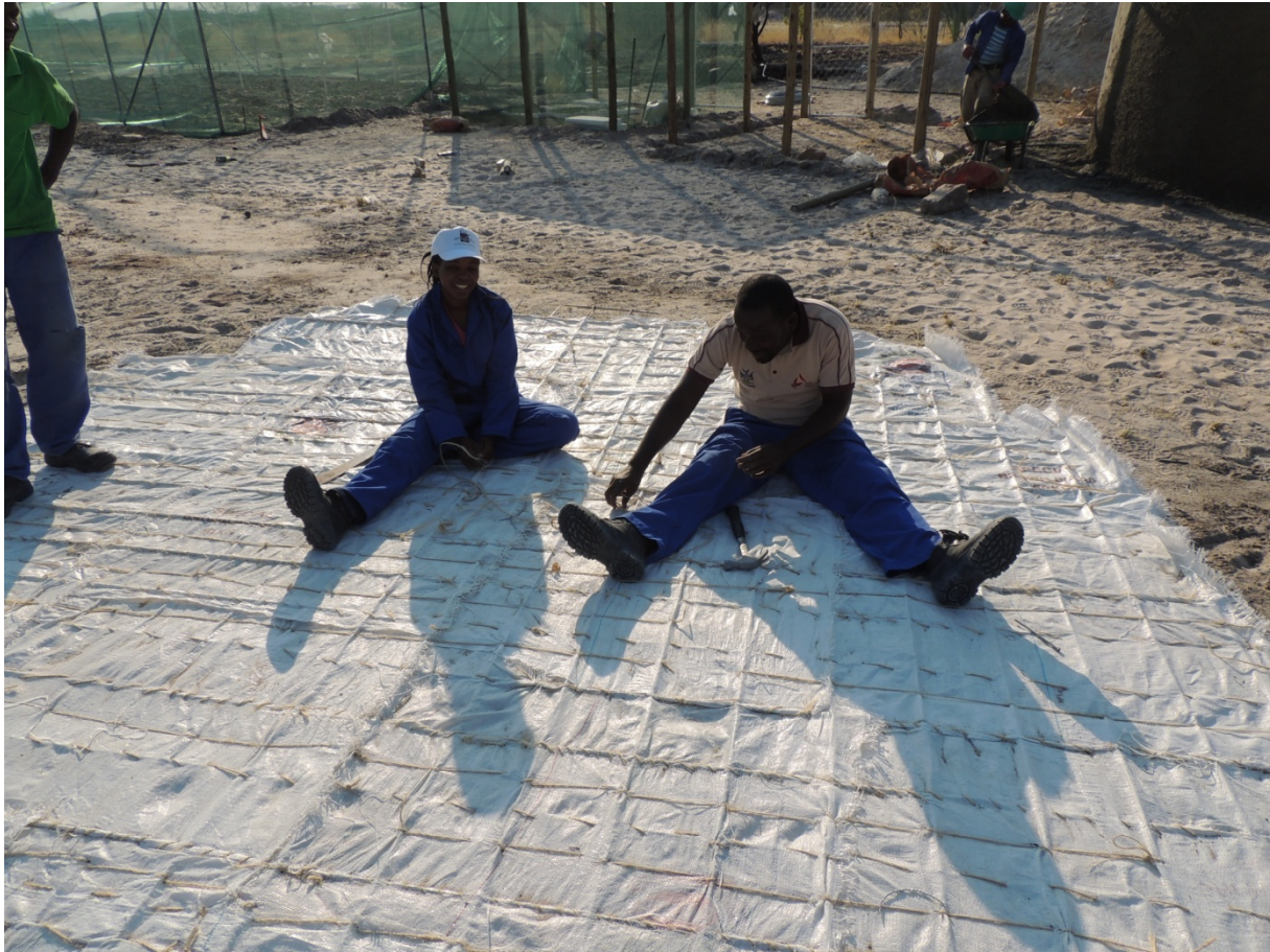
Figure 22: Tying sacks to roof reinforcement with rope and needle.
