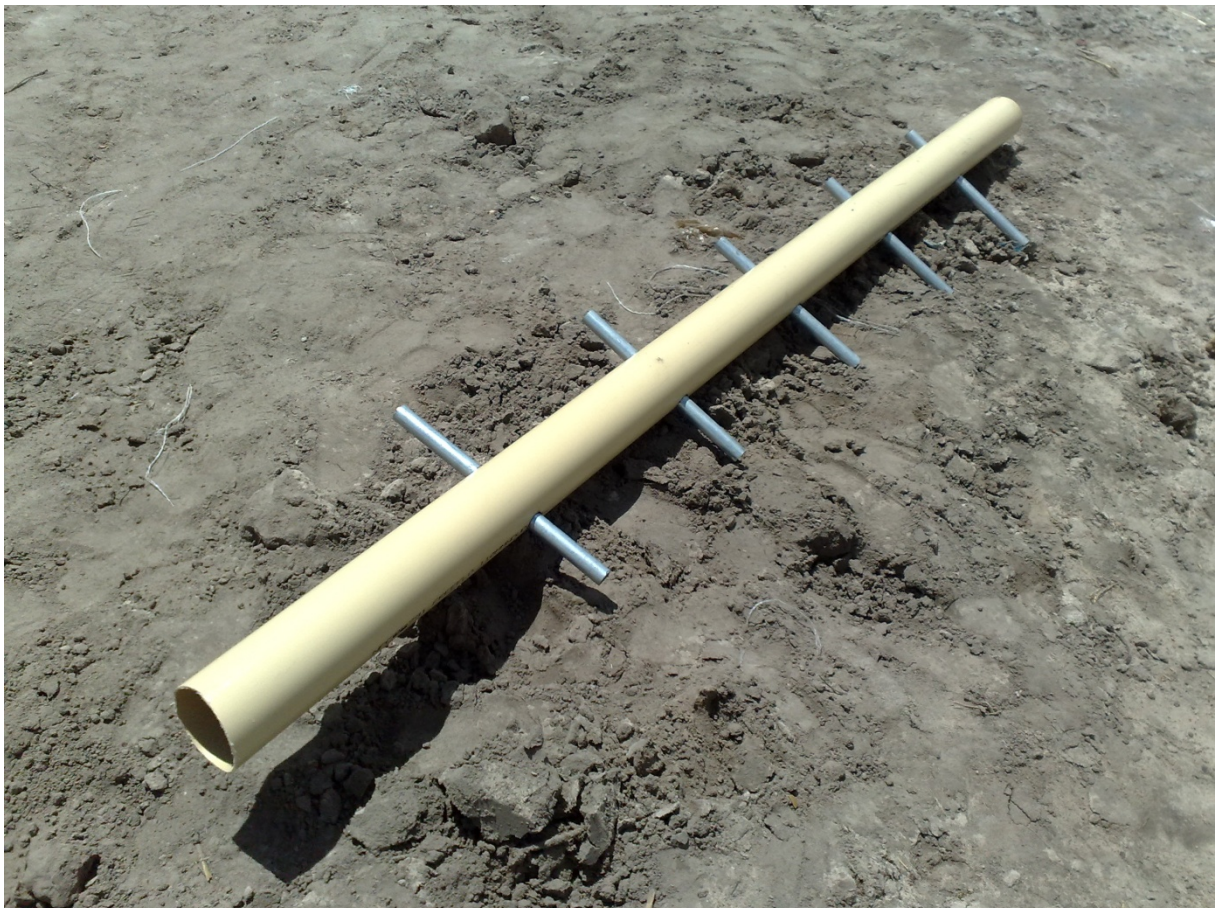
Figure 27: 4" PVC pipe with aluminum pipes assembled to it. Pipe has to be fixed to roof reinforcement near manhole and has to be filled with concrete.
