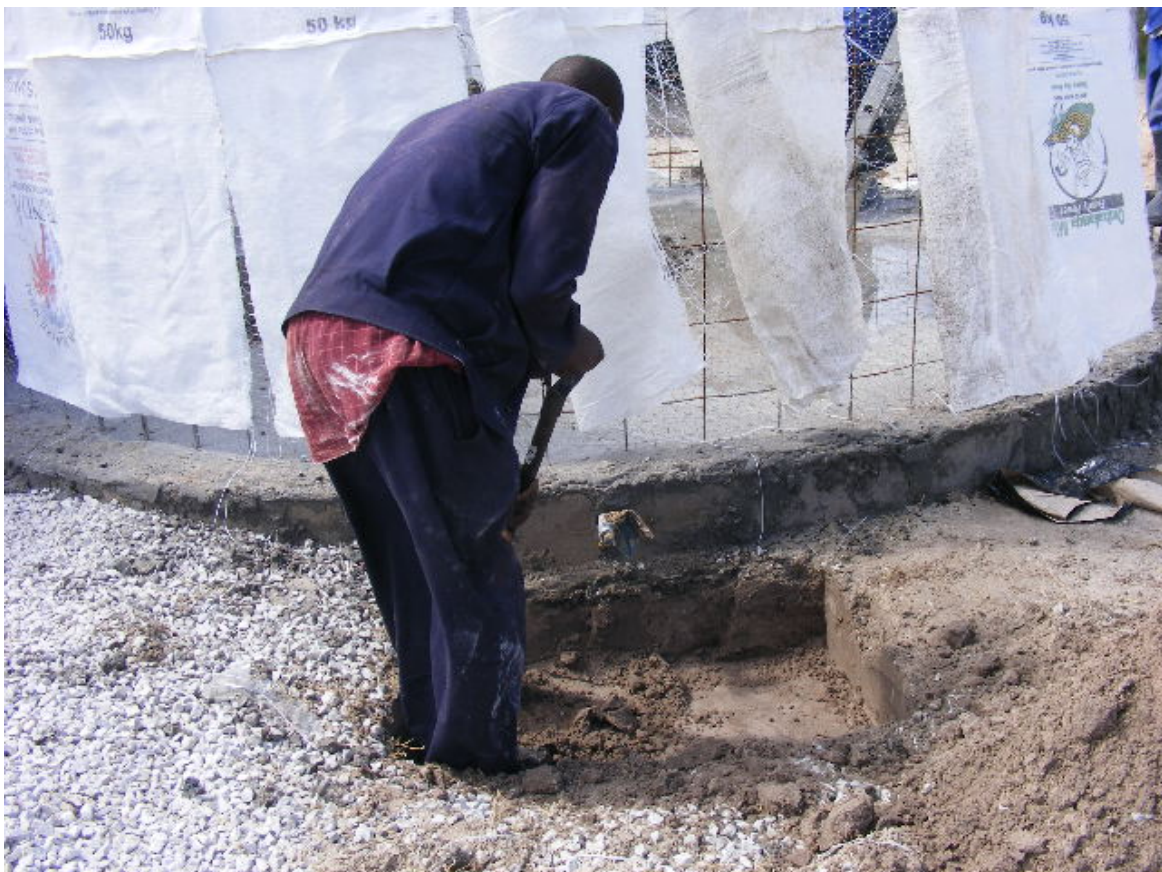
Figure 13: Excavation of future water tap pit.
