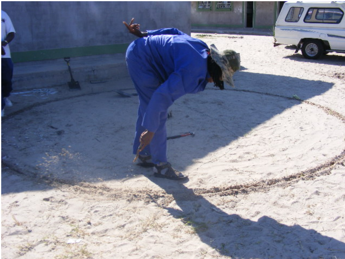
Figure 8: Drawing a circle where the foundation of the ferrocement tank shall be build.
